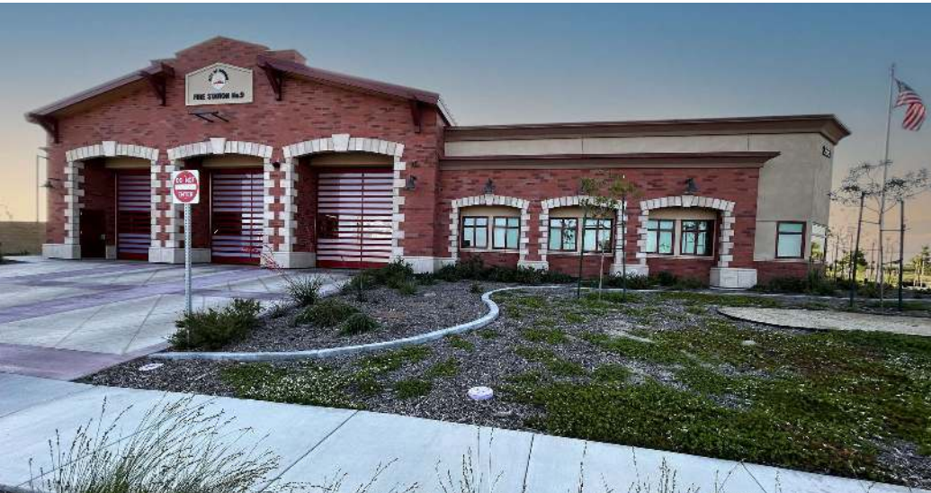
Ontario Fire Station No. 9
